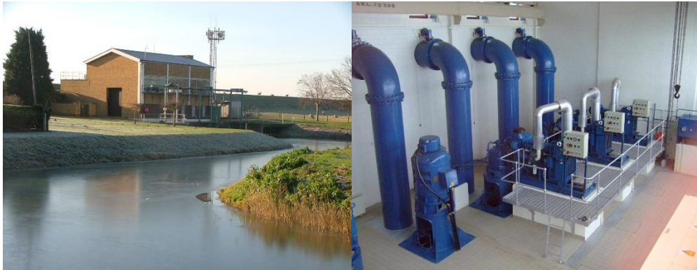
Figures 5-10 and 5-11: Cross Guns Pumping Station inside (left) and outside (right). Source: North Level District IDB
